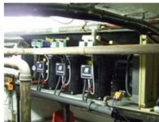
Three pumps extract heat from the ground
